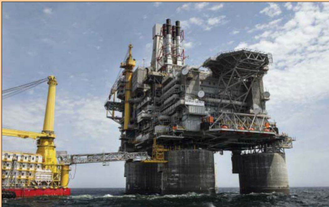
Link: the Berkut platform at the Arkutun-Dagi oilfield in Russia
